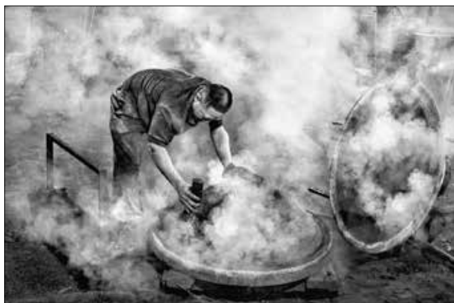
Work in heat 1
